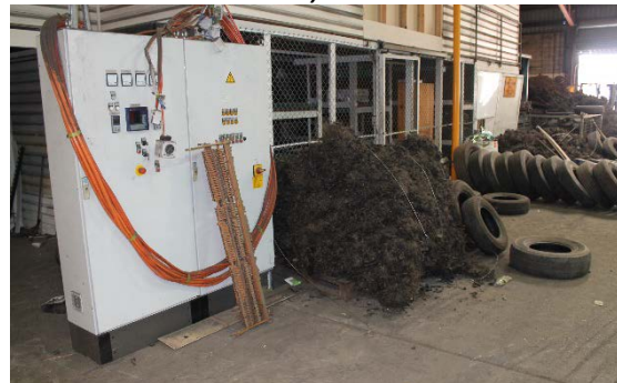
Unlicensed operators often stack tyres and waste around fire ignition points like this transformer at a western Sydney facility
