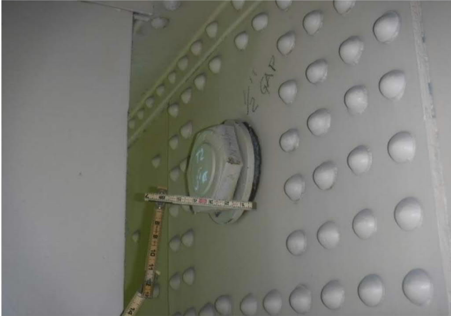
Photo 5b – Loose pin nut.
