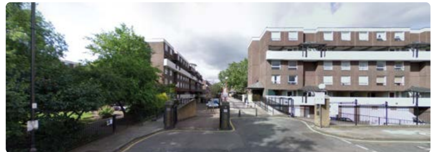
Before – Packington, Islington – Google Street View
