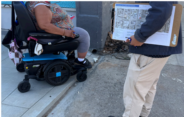
FIGURE 3: PARTICIPANTS OBSERVED MISSING CURB RAMP ALONG THE ALLEY BETWEEN HIGHLAND AVENUE AND 45TH STREET
