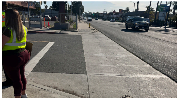
FIGURE 4. AN UNMARKED CROSSING AT E STREET AND JEFFERSON AVENUE WHICH WAS NOTED TO BE MISSING A YELLOW CROSSWALK AS IT IS NEXT TO THE SCHOOL
