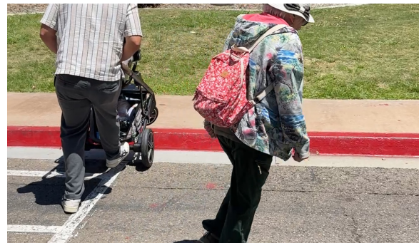
FIGURE 4: PARTICIPANTS OBSERVED A MISSING CURB RAMP NEAR ALCAZAR PARKING LOT'S SIDEWALK.
