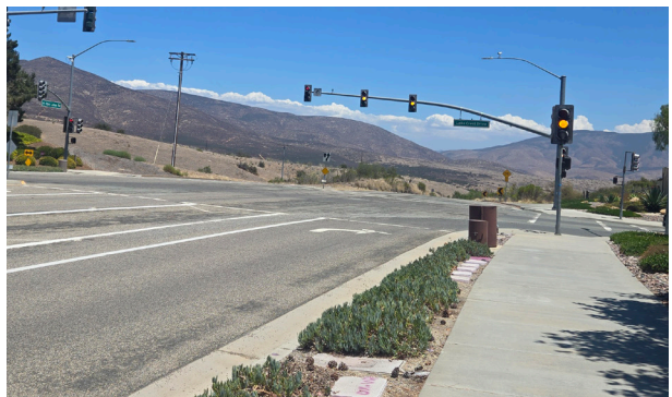
FIGURE 4: DESPITE CLASS II BIKE LANES AND SHARROWS ON OTAY LAKES ROAD, THE 50 MPH SPEED LIMIT AND LACK OF PROTECTION LEADS CYCLISTS TO RIDE ON THE SIDEWALK.
