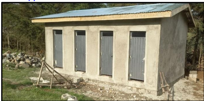
A completed latrine at Edoy Elementary
