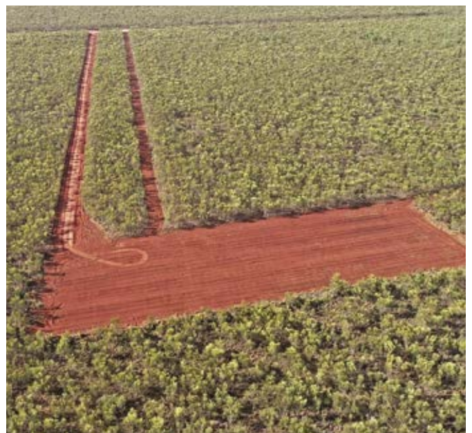
Landclearing of Bilby habitat in Broome by the Water Corporation
