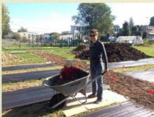
Building the farm in 2013
