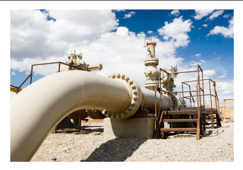
Each main line valve site would comprise the following components located within a fenced compound; above ground pipework and automated mainline isolation valve with gas over oil actuator, pipeline blowdown vent, remote terminal unit, self-contained solar power supply and satellite communications, cathodic protection unit, ground bed and test points
