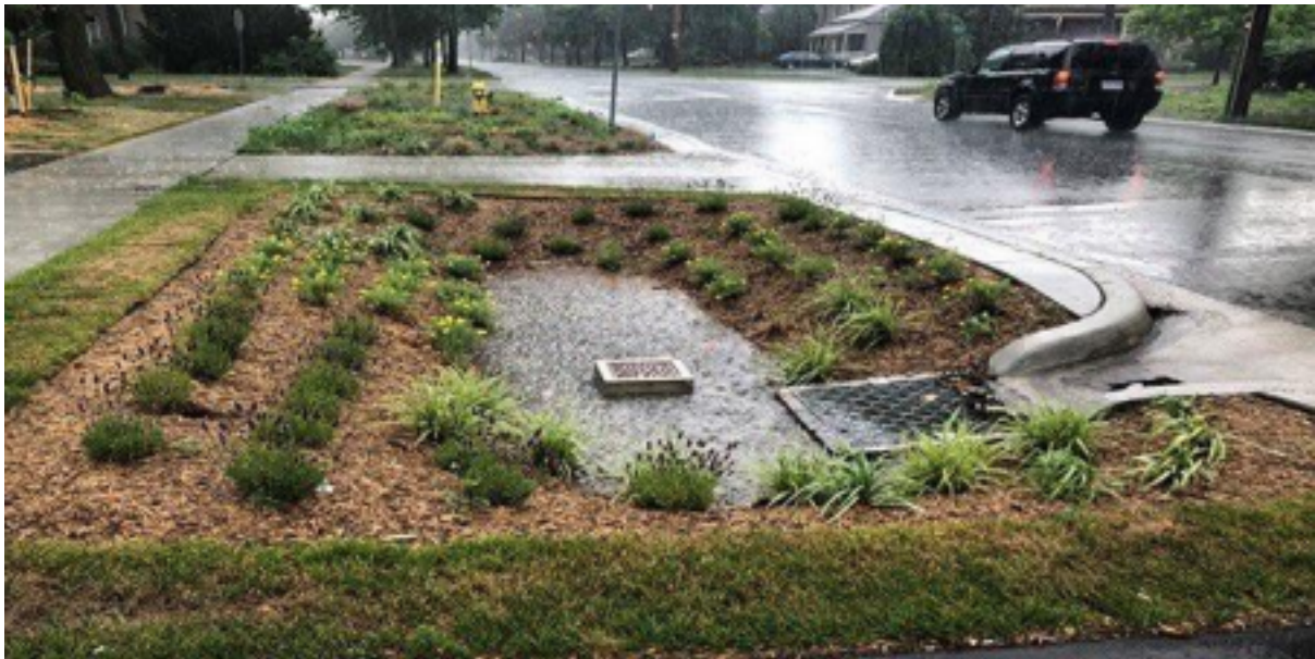
Photo of a rain garden. Source: City of London
