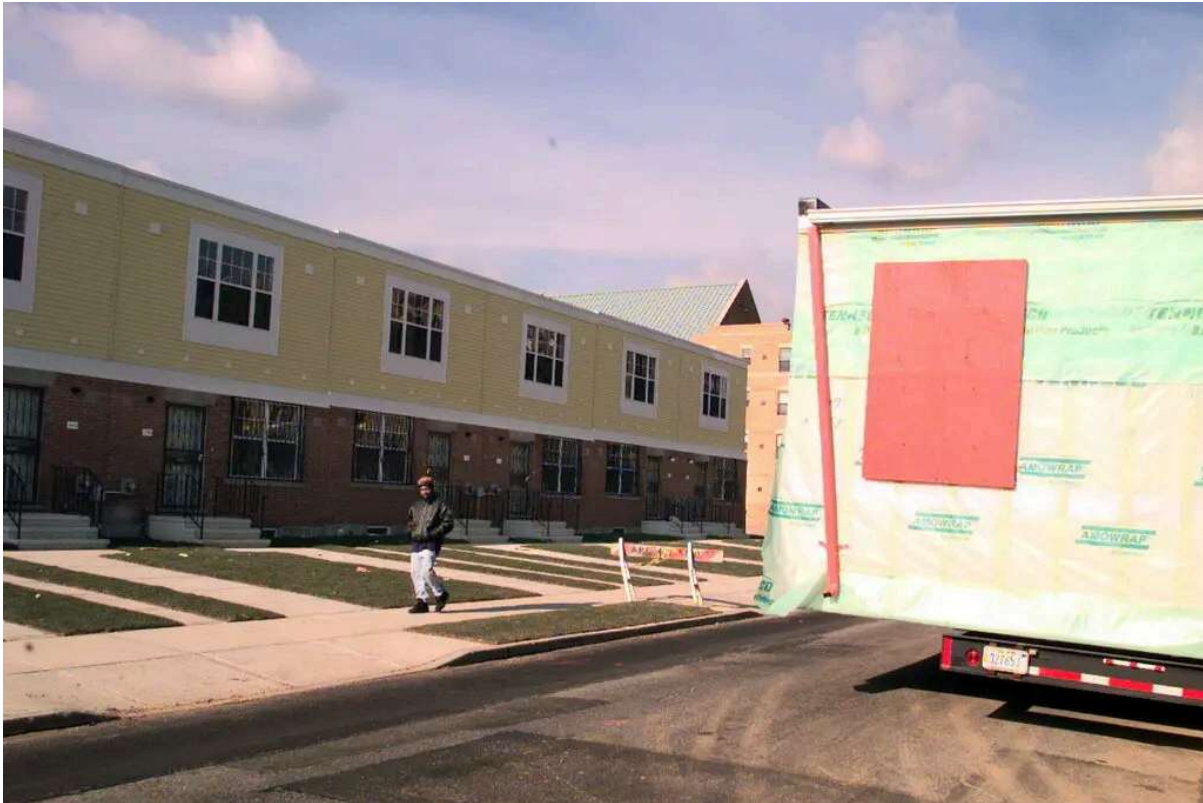
Prefabricated portions of some early Nehemiah homes were delivered on trailers to plots of land in East New York in 1997. Andrea Mohin/The New York Times
