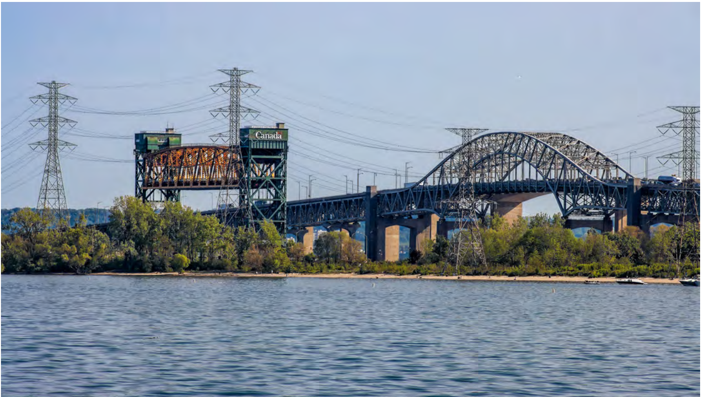
Burlington Canal Lift Bridge. STOCK PHOTO
