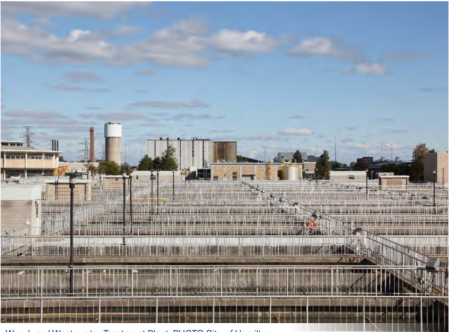
Woodward Wastewater Treatment Plant. PHOTO City of Hamilton
