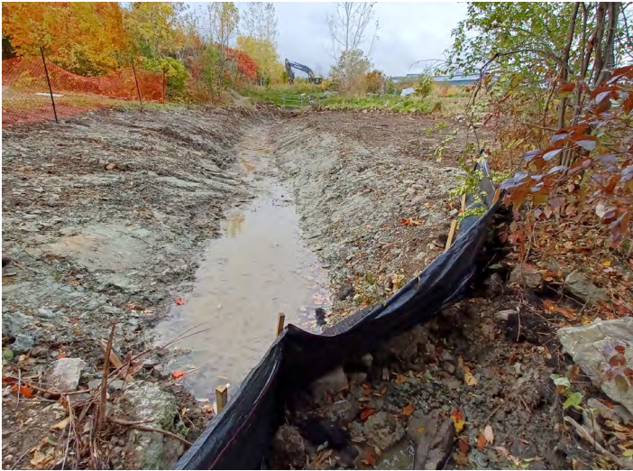
Sediment Control Fencing. PHOTO City of Hamilton
