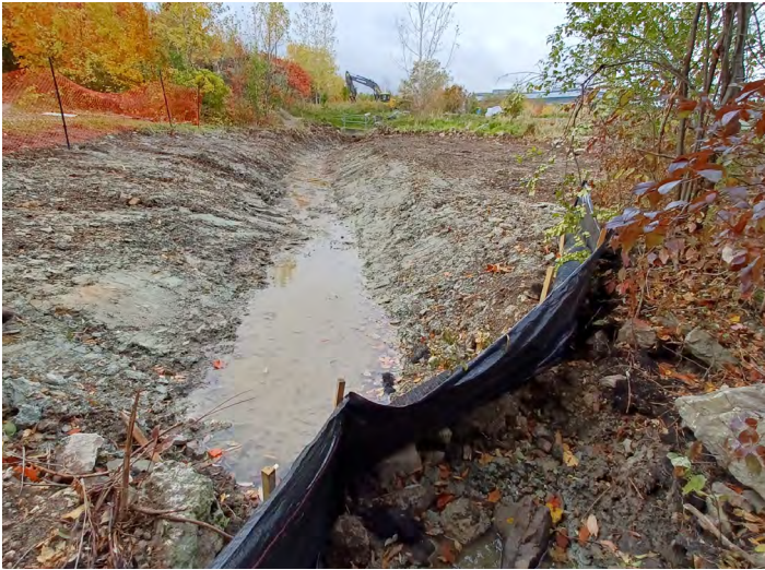
Sediment Control Fencing. PHOTO City of Hamilton
