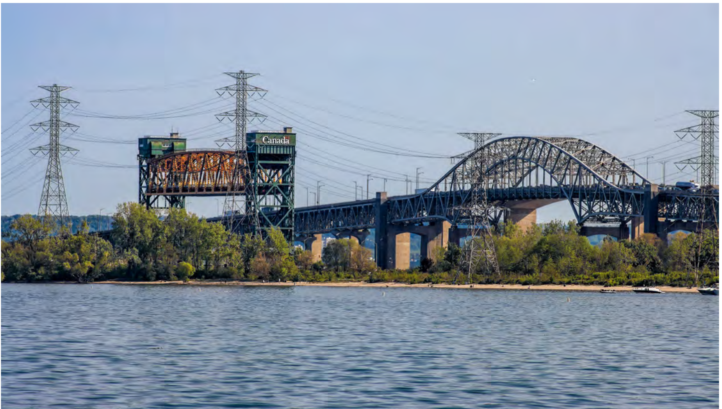
Burlington Canal Lift Bridge. STOCK PHOTO
