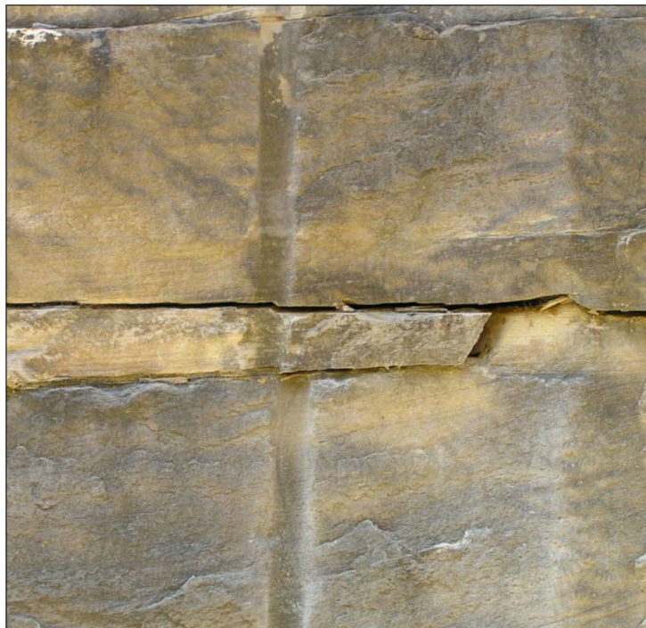
Figure 6. Vertical rock cutting showing mining-induced basal shear plane formation along bedding sub-horizontal bedding planes in the Southern Coalfields (reproduced from SCT, 2015).
