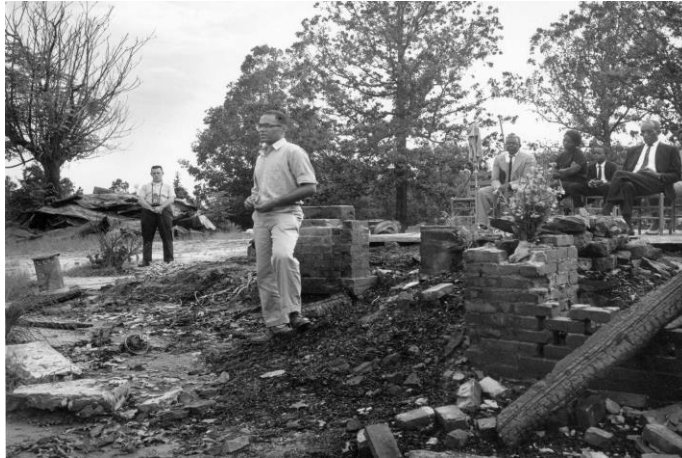
Burned ruins of the Mt. Zion Methodist Church in Neshoba County, Mississippi. Credit: Tamio Wakayama/Take Stock/TopFoto
