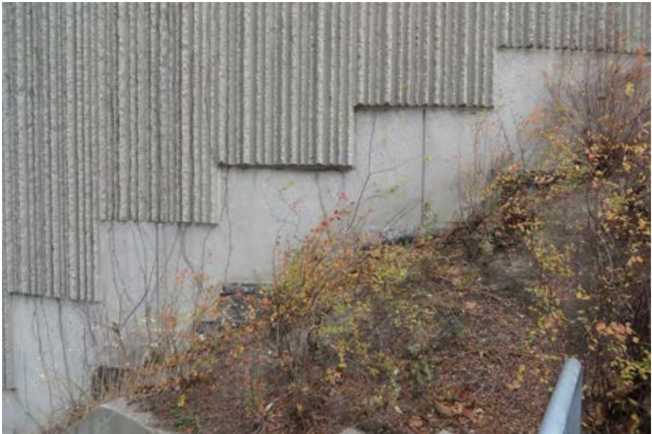
Figure 65: Detail of Core Building Tower where two concrete textures are used
