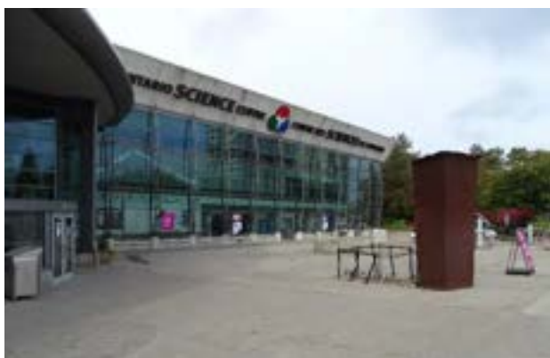
Figure 33: View north toward Omnimax
