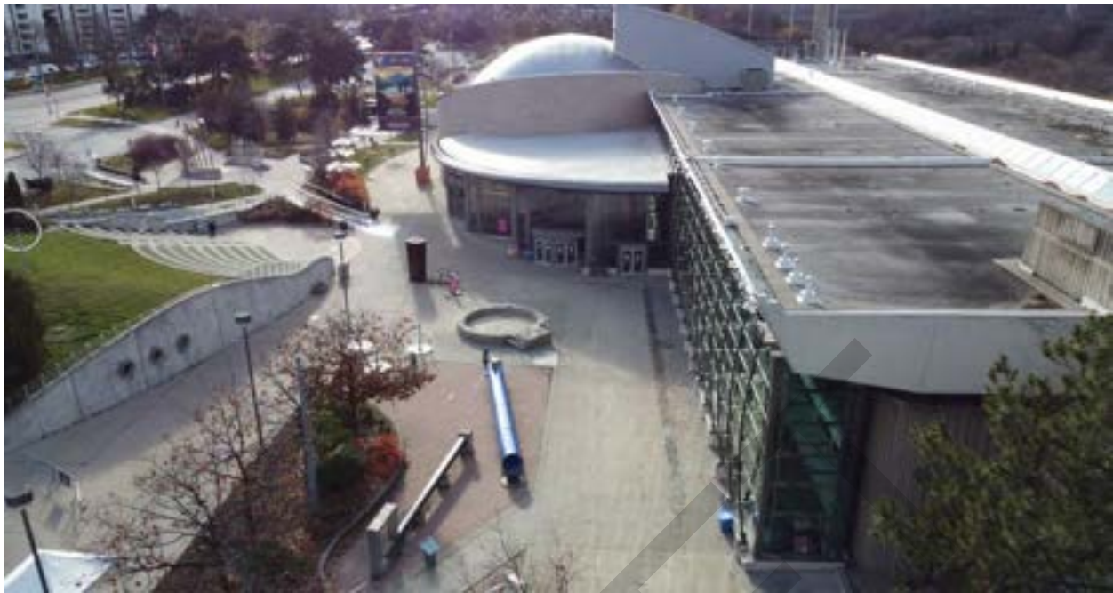
Figure 42: Aerial view looking south over current forecourt area
