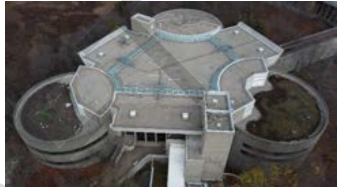
Figure 61: Roof of the Core Building with the Green Roof visible
