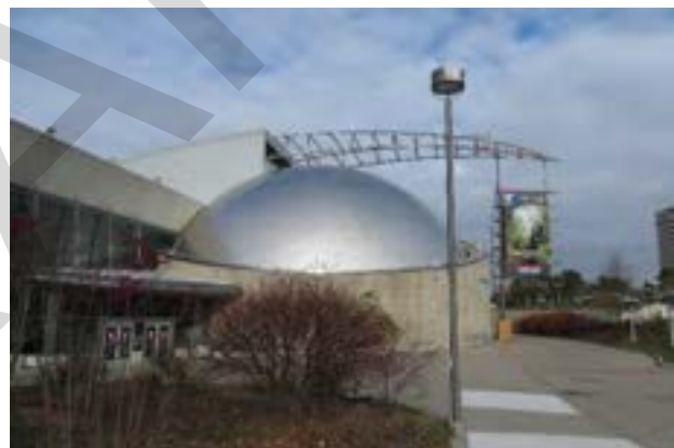
Figure 35: Main Entrance forecourt space
