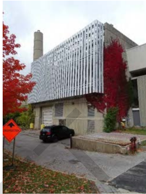
Figure 78: View of the exterior of the Boiler Plant at south side of Main Entrance Building
