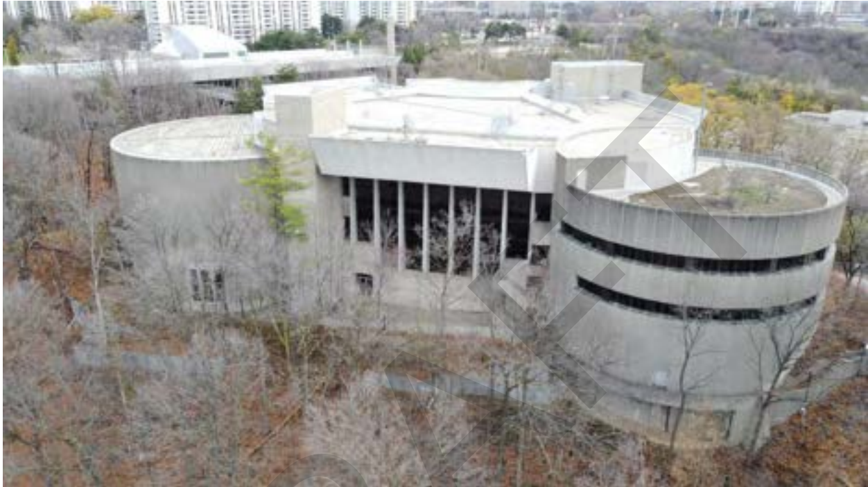
Figure 92: Southwest façade of Core Building
