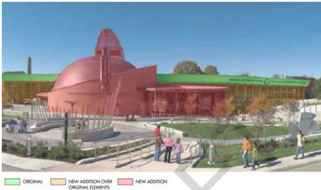
Figure 23: Main Entrance primary elevation c. 1996 Credit: Ontario Science Centre with SBA annotation
