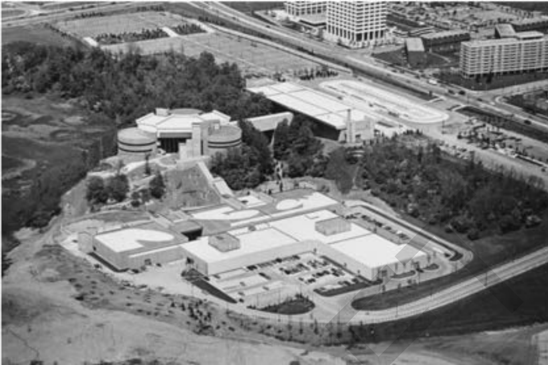
Figure 20: Aerial view looking northeast. c. 1969 (Credit: City of Toronto Archives Series 1745, File 9, Item 5)
