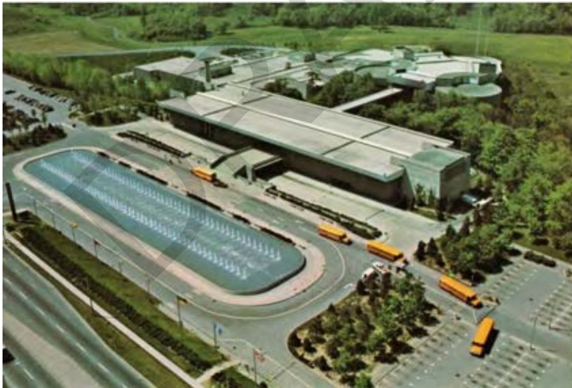
Figure 21: Original Main Entrance with forecourt fountain c. 1970 (Credit: Moriyama & Teshima Architects)
