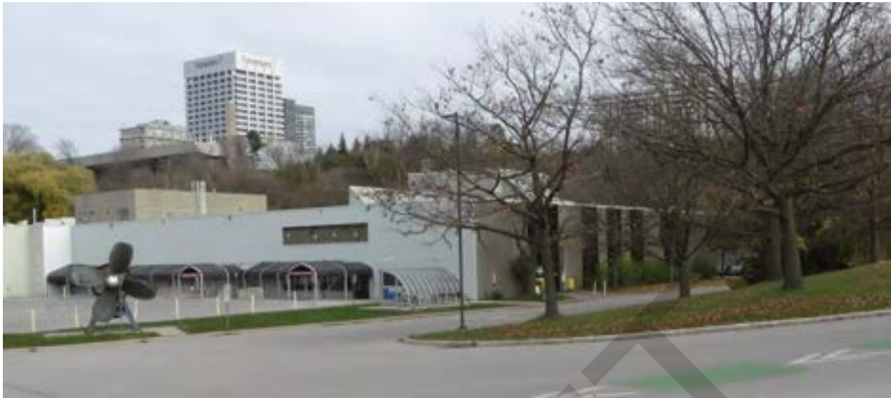
Figure 115: Southwest façade of Valley building with security/visitor entrance
