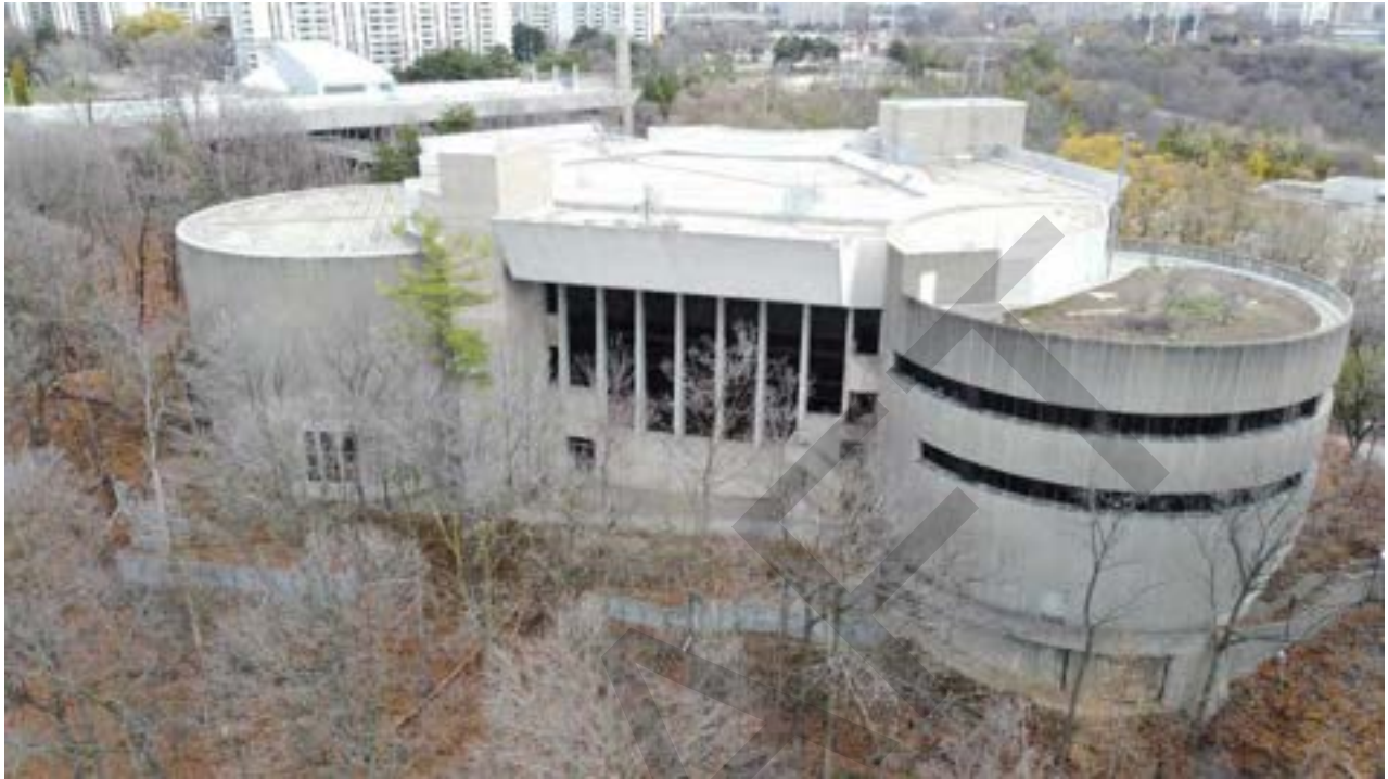
Figure 68: View of West side of Core Building with prominent windows overlooking ravine
