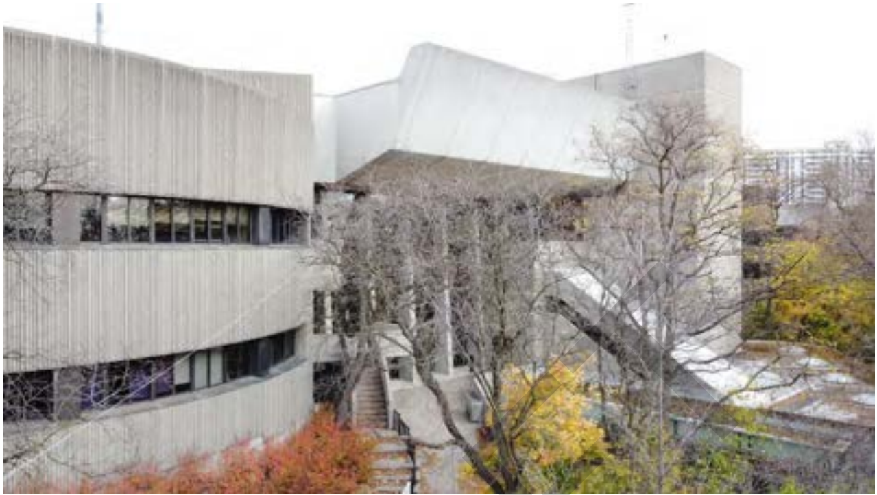
Figure 93: West facade of Core Building facing the ravine
