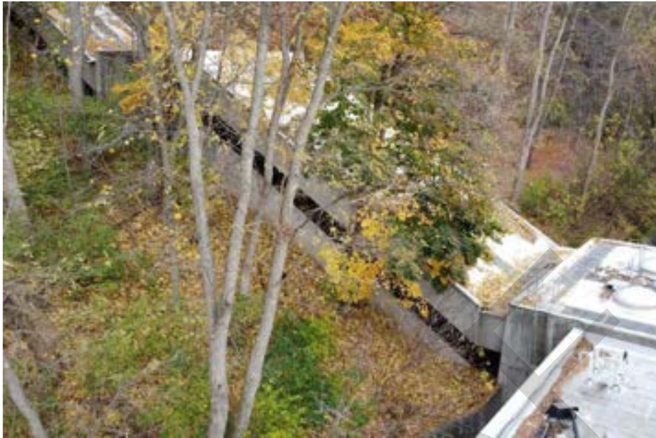
Figure 49: Exterior view of escalators
