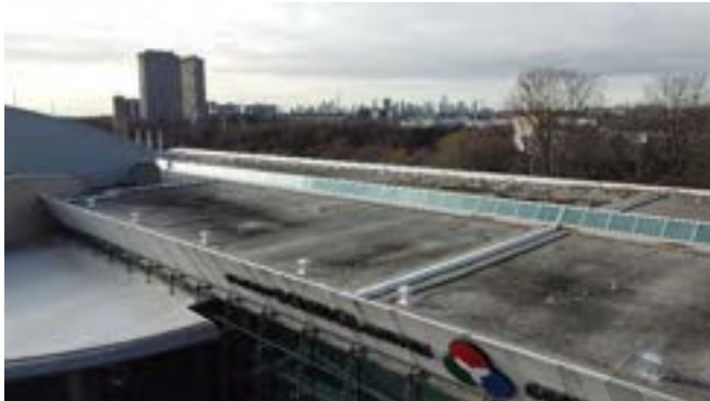
Figure 62: Roof of Main Entrance Building with row of skylights visible
