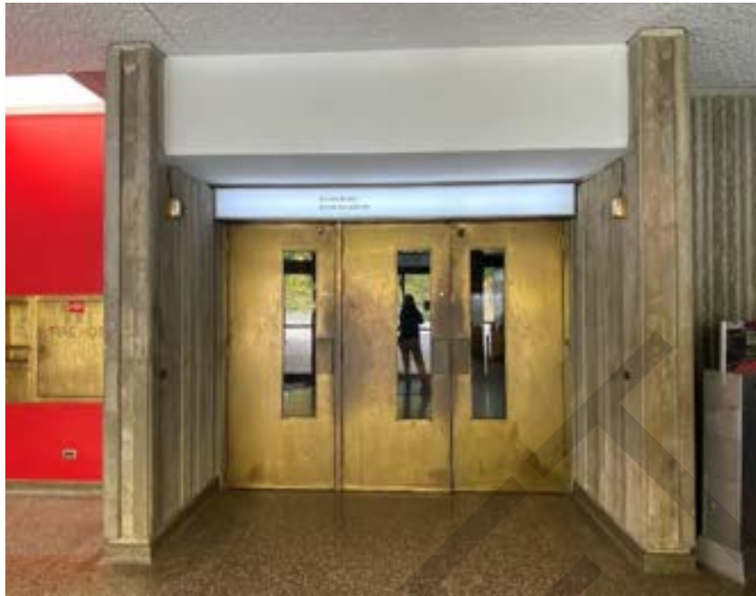
Figure 74: Entrance to Discovery Exhibition Space with brass doors and door pulls
