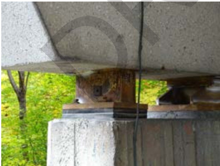
Figure 48: Detail of connection point on pier supporting bridge
