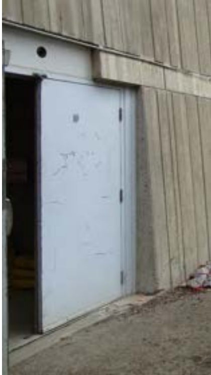
Figure 71: Exterior Metal Door on West Elevation of Main Entrance Building
