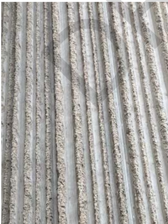
Figure 66: Detail of concrete texture prevalent throughout complex
