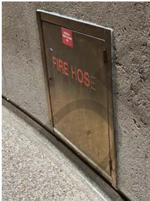
Figure 76: Brass door on fire house cabinet in Core Building
