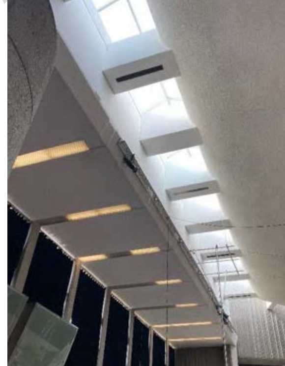
Figure 107: Skylights in the central exhibition space
