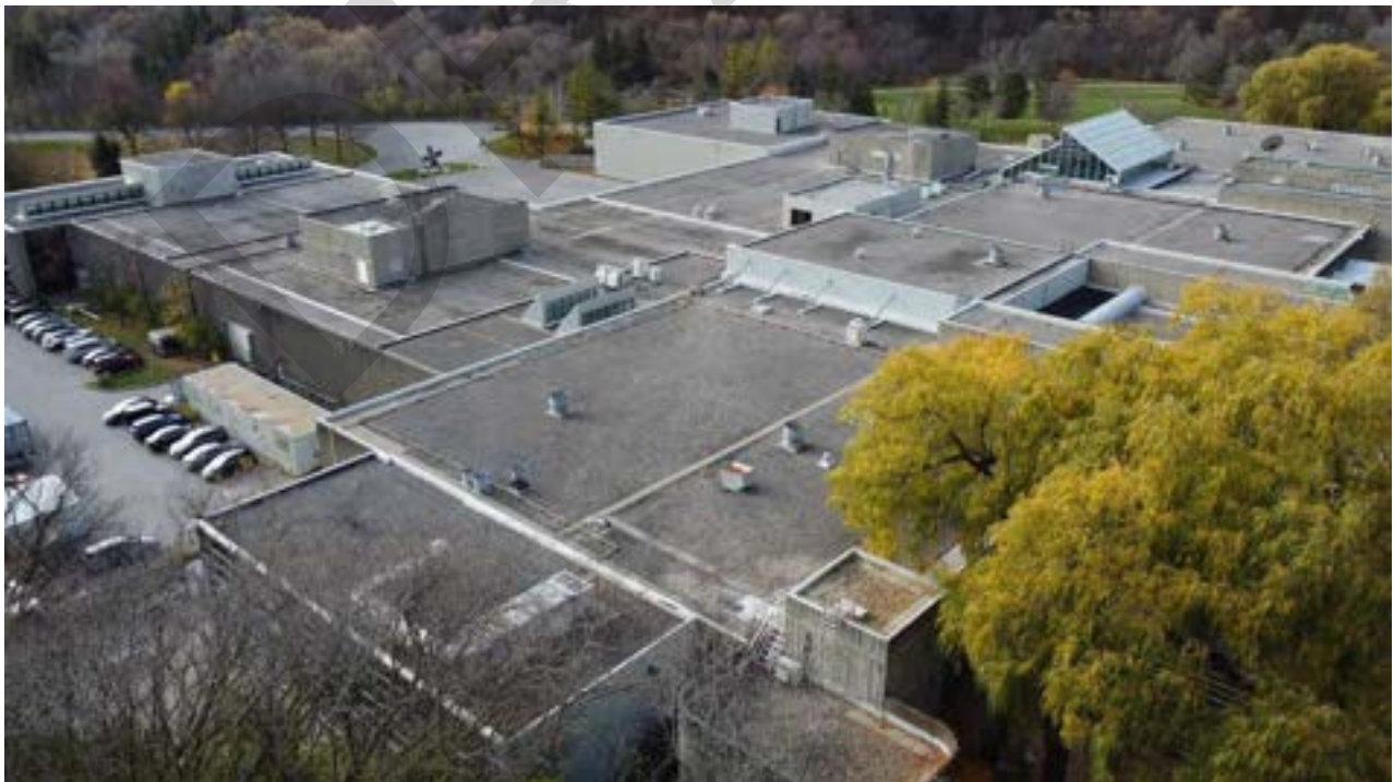
Figure 113: View southwest of the Valley Building
