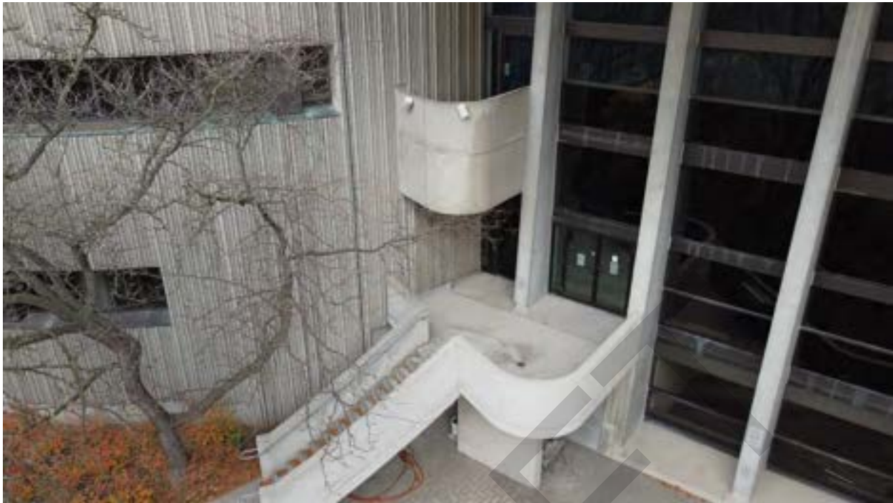
Figure 98: Exterior Stair on west side of Core Building leading to upper level, pedestrian path and upper balcony
