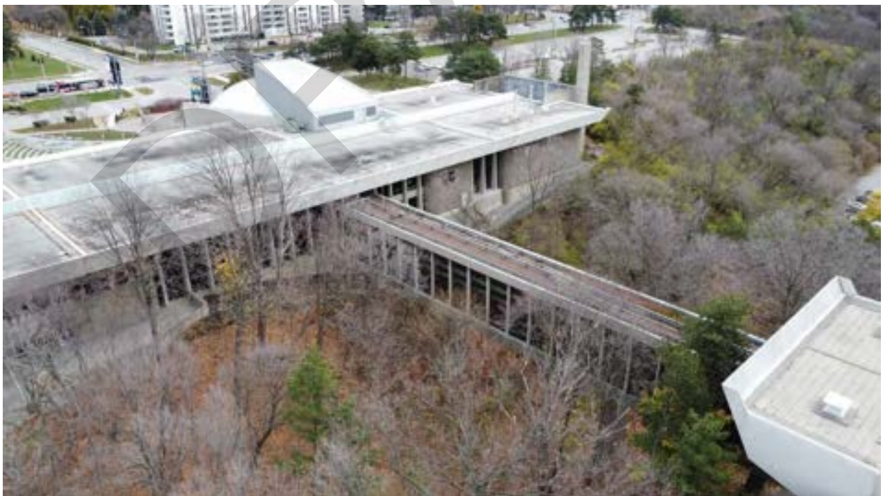
Figure 69: View northeast where windows on the bridge and the west elevation of the Main Entrance Building are visible
