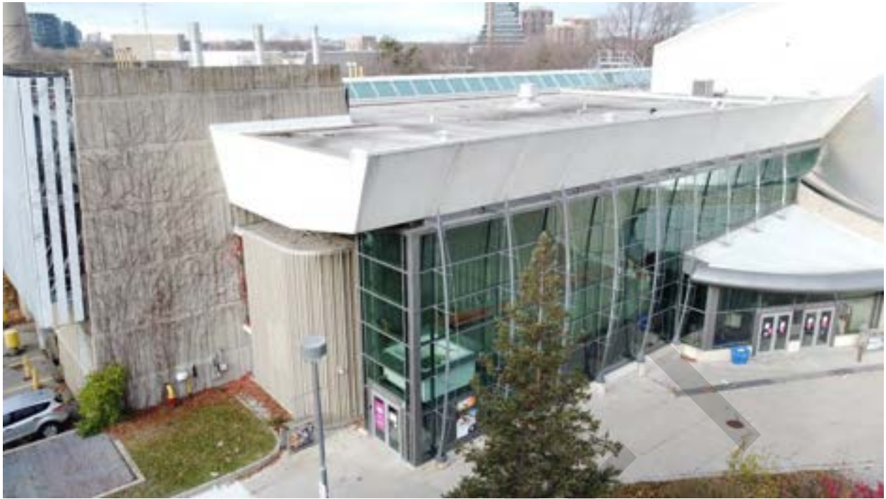
Figure 91: Glazed group entrance
