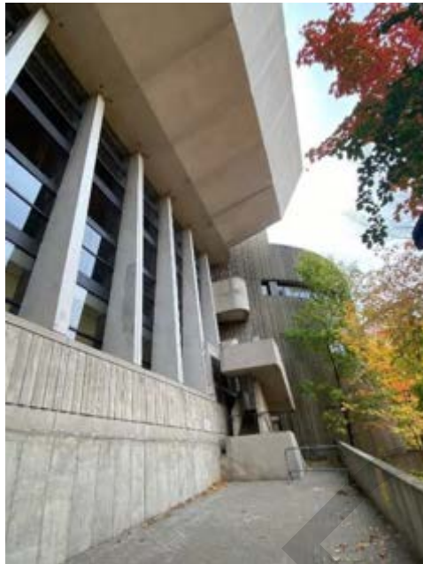
Figure 96: Large windows looking west towards the TRCA lands
