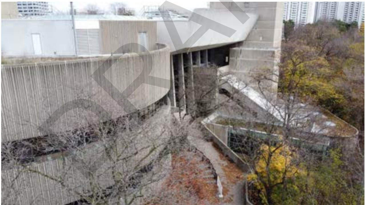
Figure 28: Aerial view looking at the west side of Core Building
