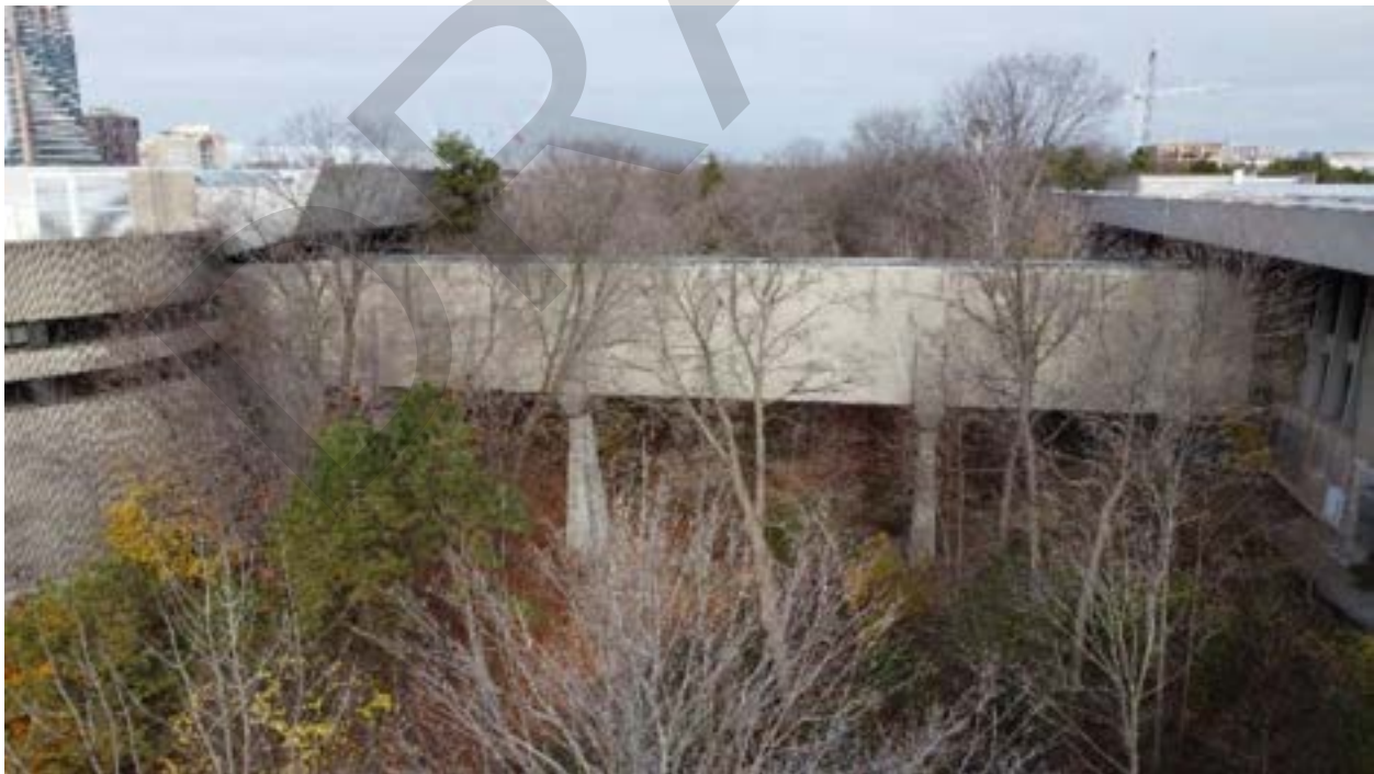
Figure 46: South side of Bridge
