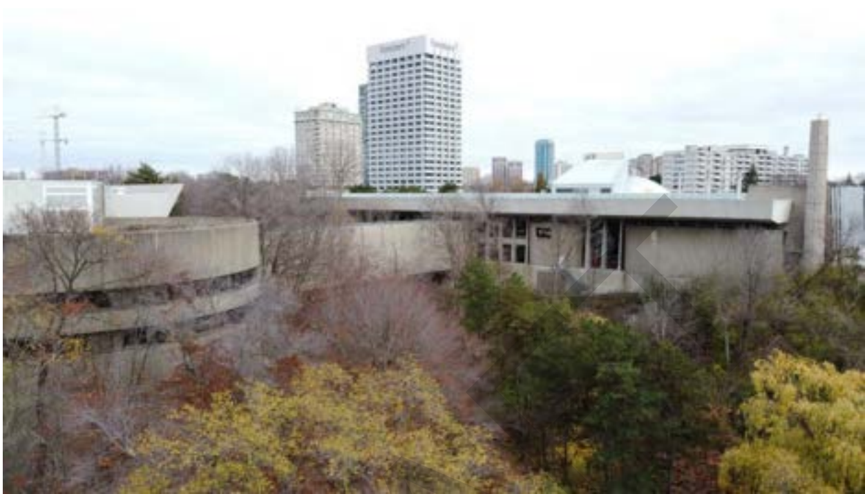
Figure 25: View northeast with rear of Main Entrance to right of image, bridge, and Core Building in view
