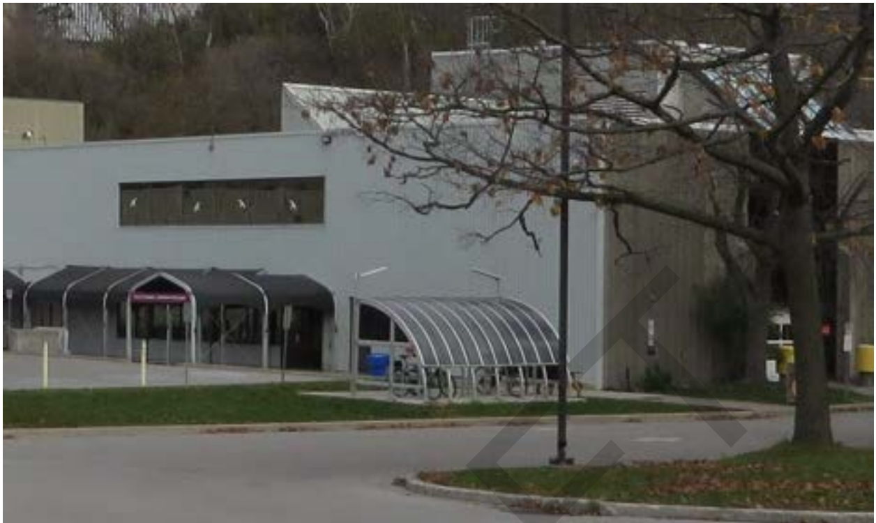
Figure 67: View of Valley Building's southeast wing where both concrete and vertical paneling was used
