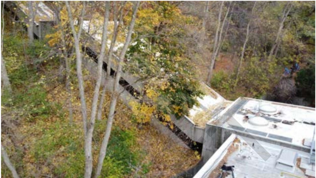
Figure 29: View of Escalators connecting Core Building (to right of image) with Valley Building set into the natural ravine embankment
