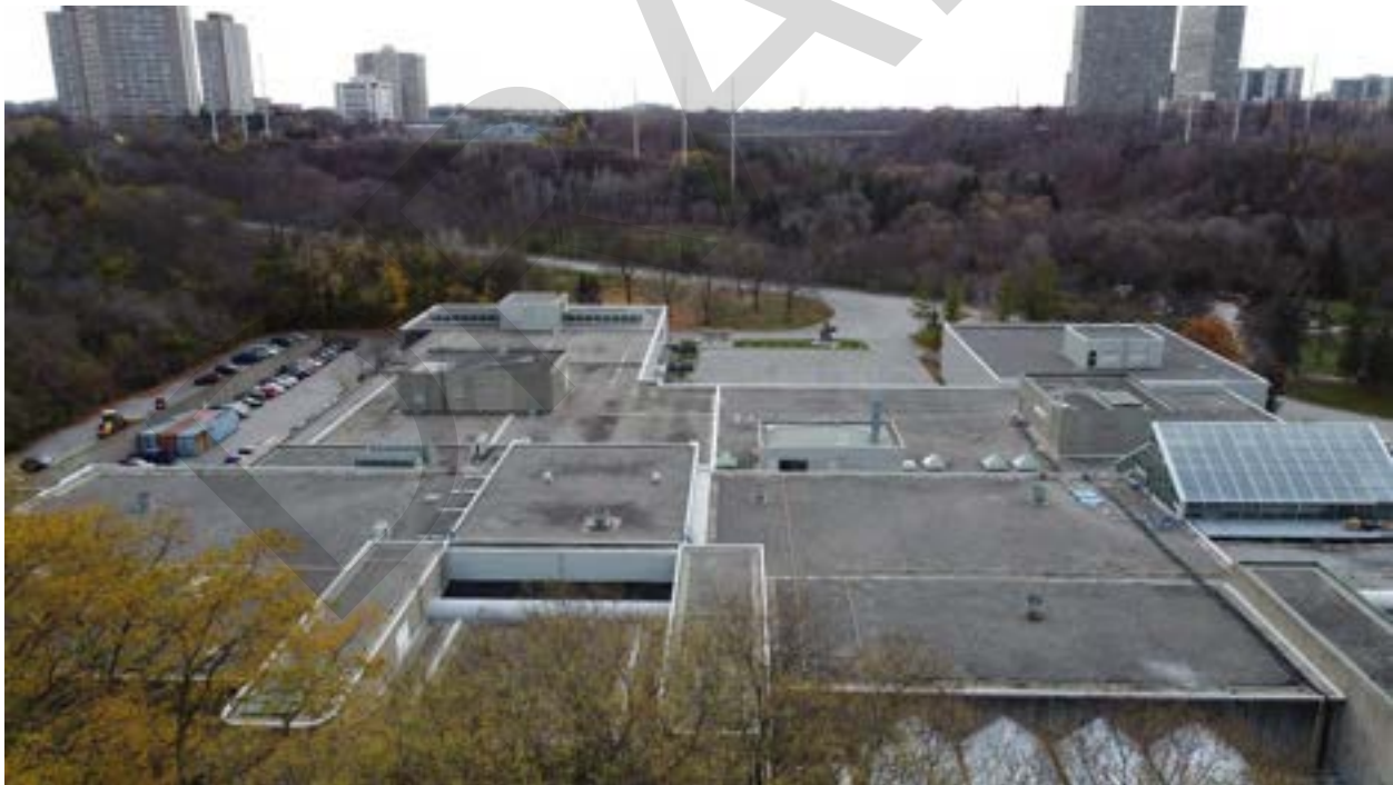
Figure 118: Aerial looking south over Valley Building Roof
