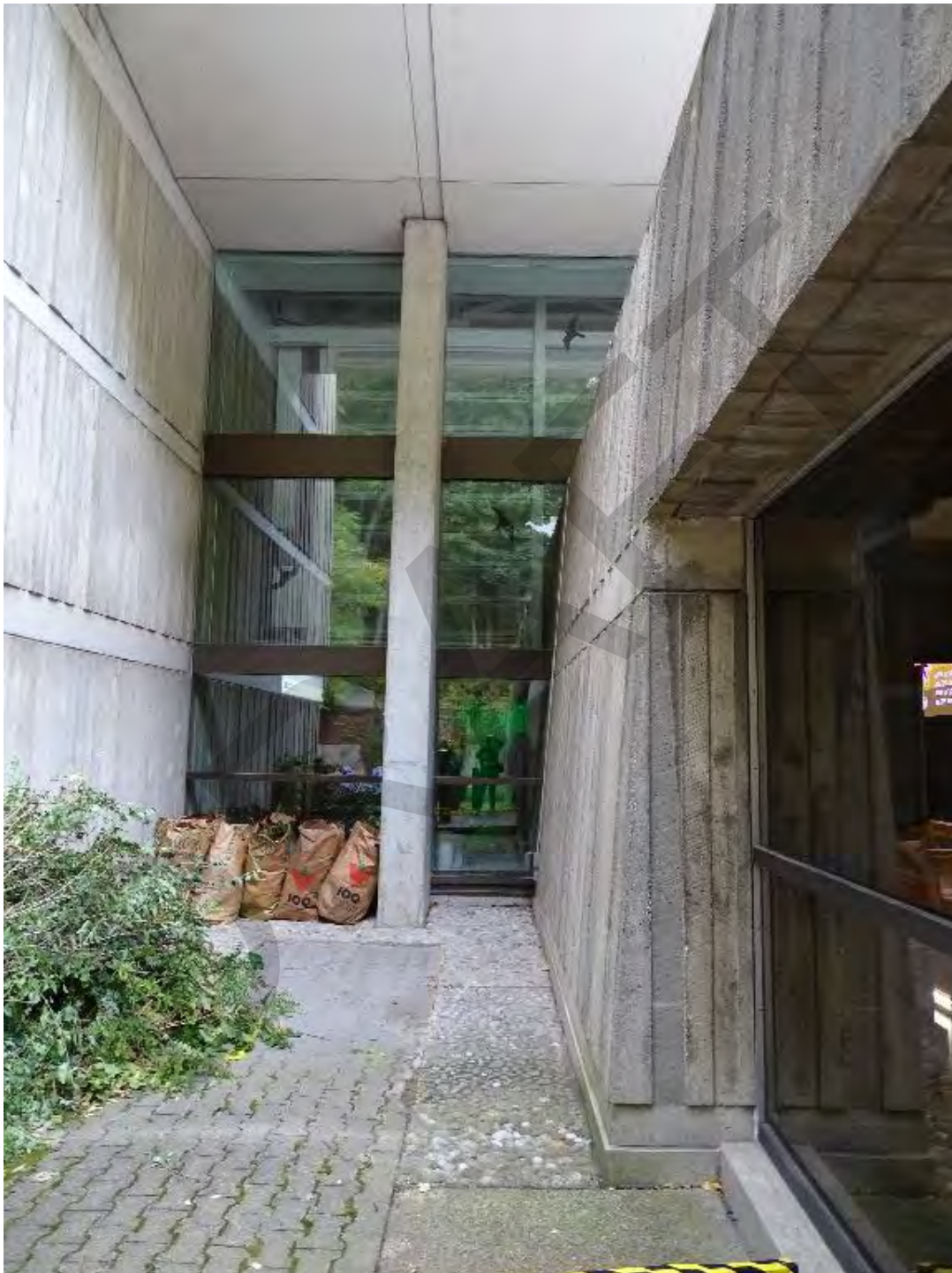
Figure 70: Windows in Valley Building where storefront system visible
