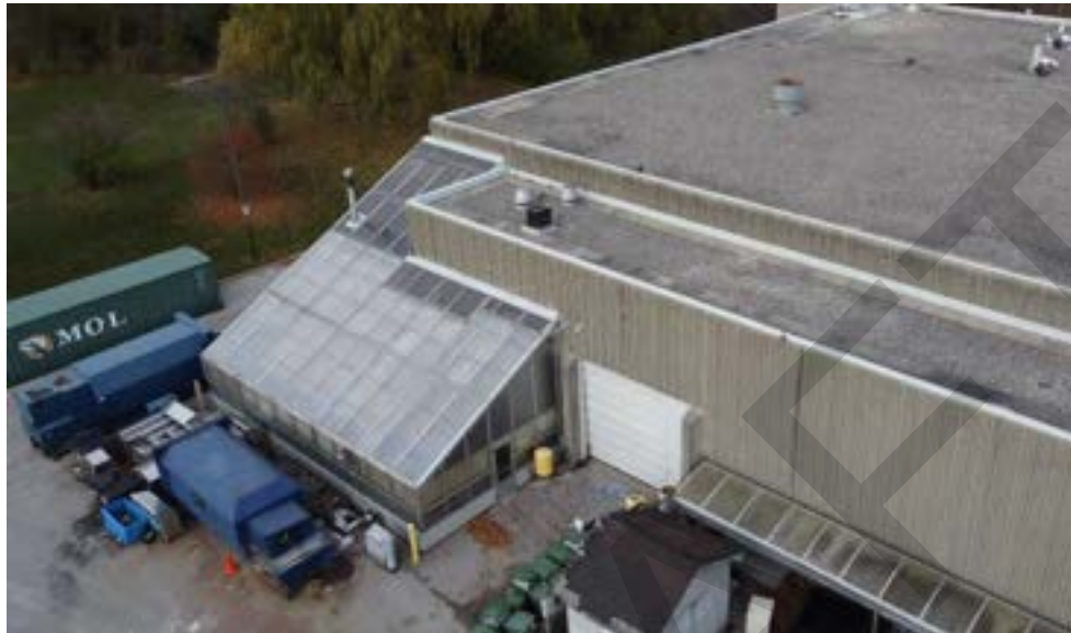
Figure 133: Greenhouse addition on southwest corner
