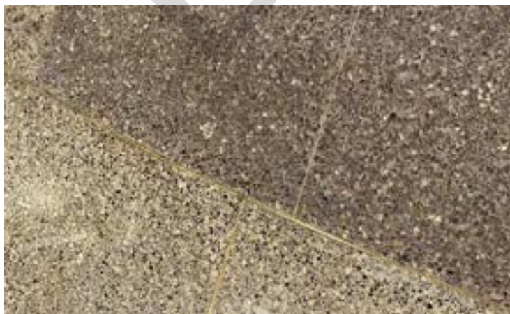
Figure 73: Terrazzo floor with bronze divider strips
