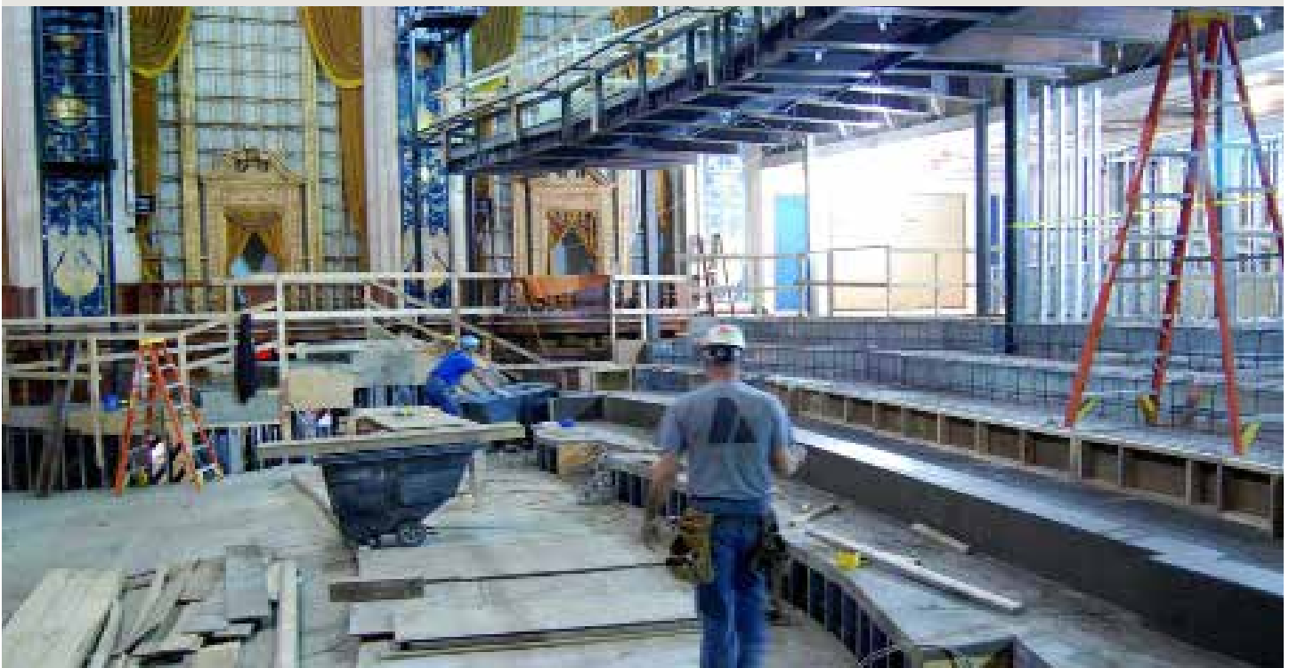
Allen Theater Renovations (Photo: Tony Brown, The Plain Dealer)
