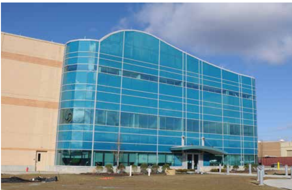
NEORS D Southerly Waste Water Treatment Plant - Renewable Energy Facility
