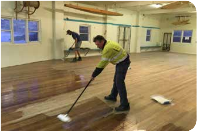
Denis in action resurfacing the hall floor
