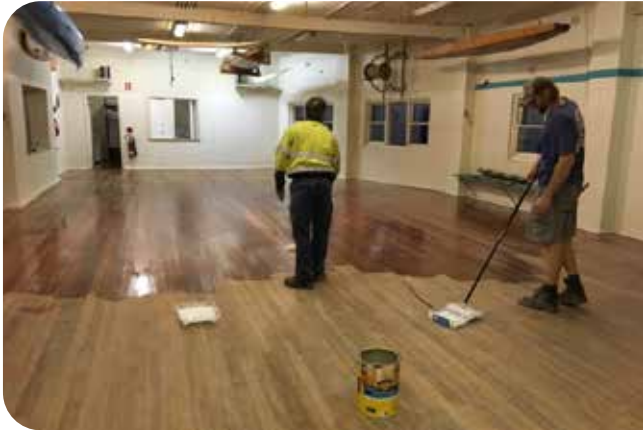
Resurfacing the hall floor
