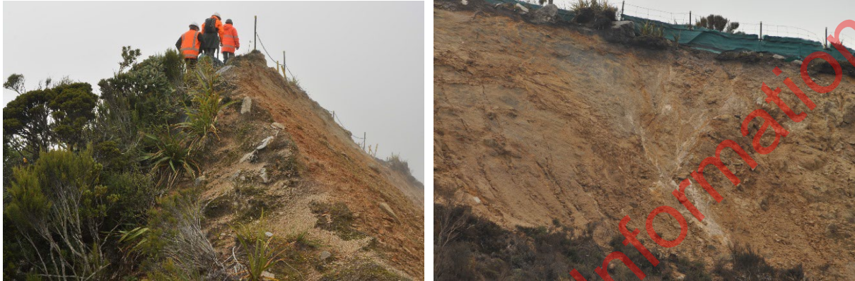
Figure 7. The steep, eroding eastern side of NASA after coal extraction. The slope was left over-steepened, leading to erosion of the best remaining natural habitat of P. augusta on the adjacent DOC land to the west.
