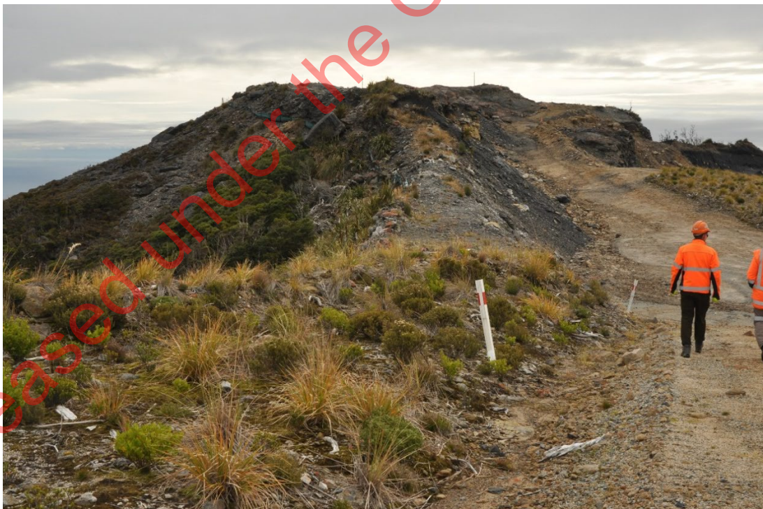
Figure 4. The road along the A12 ridgeline presents a barrier to snails. It needs to be retired and densely planted (once revegetation on the high point of the ridge is complete). Existing plantings on the road verges and to the east need high-density enrichment planting with appropriate native species.
