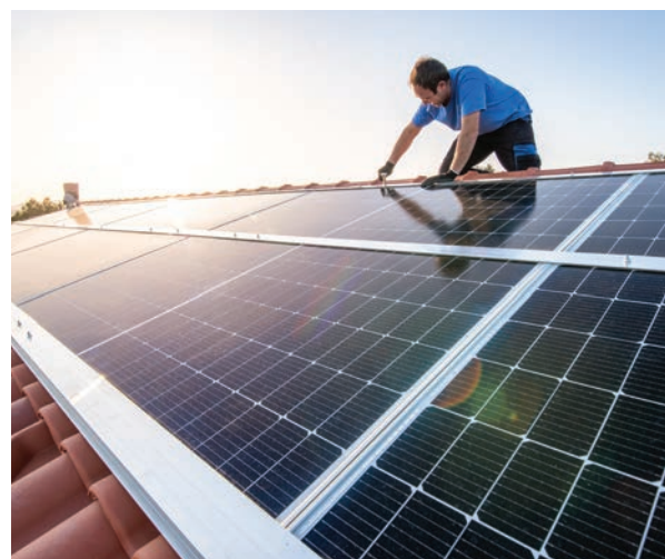
Photo: Installing solar panels – Eloï Omella – iStock
