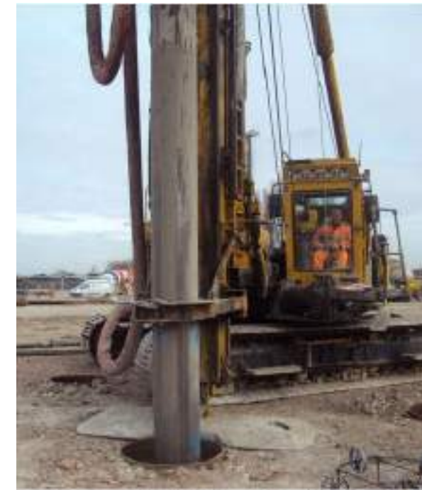
Figure 20: Example of Pile Boring with temporary casing
