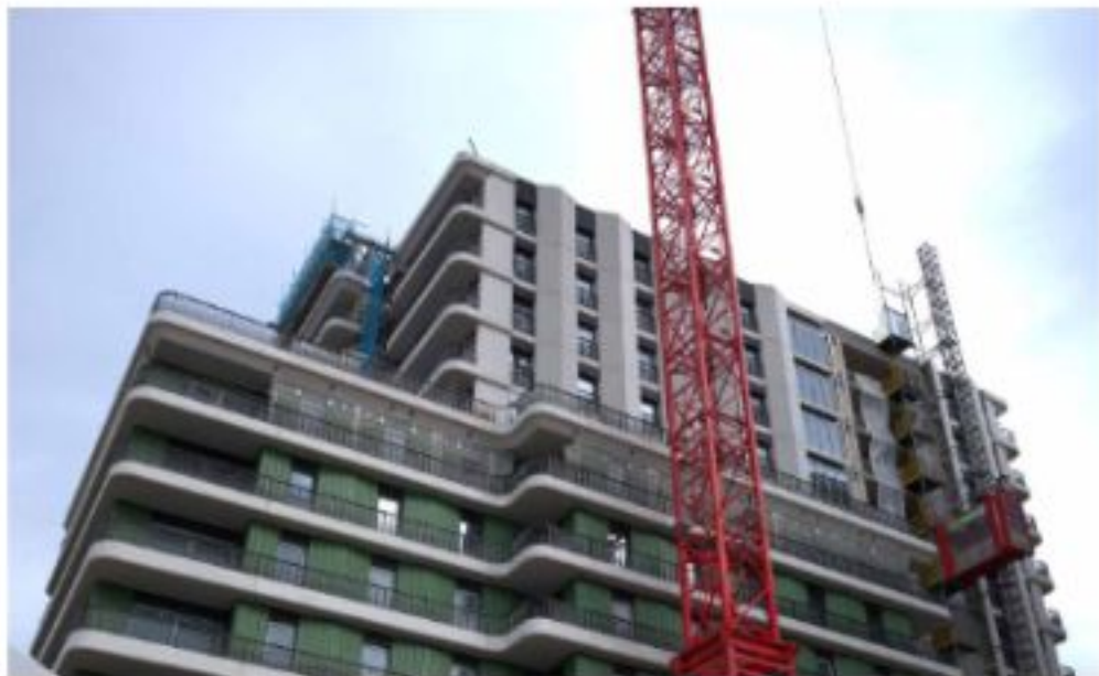
Above: Photograph from site, showing the upper levels of Building 7 as viewed from the new public square. This photo shows many of the same design principles as seen on Buildings 5 and 6. The photo again highlights the importance of high quality precast concrete soffits to all balconies and to the precast concrete perimeter feature banding.
