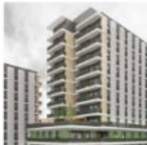
View from West (Building 5)
