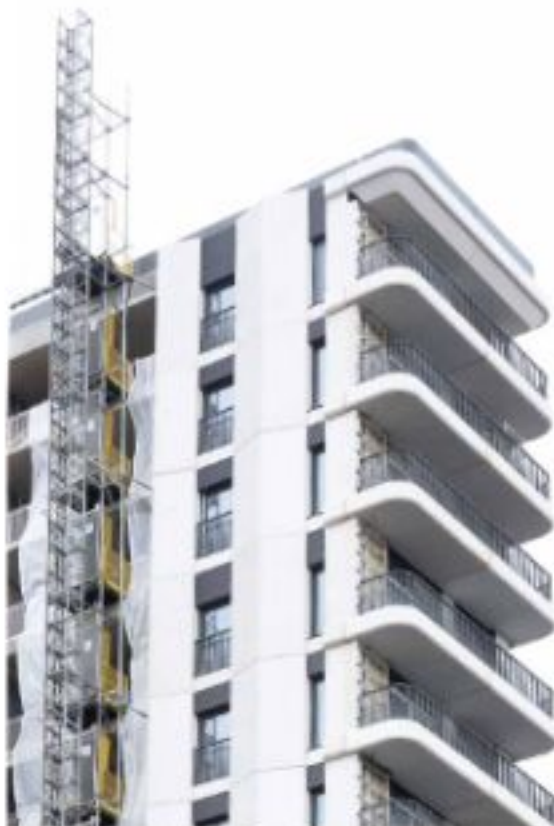
Above - photograph from site of the railway facade under construction (terracotta panels not yet installed). The photo demonstrates the importance of high quality balcony undersides.
