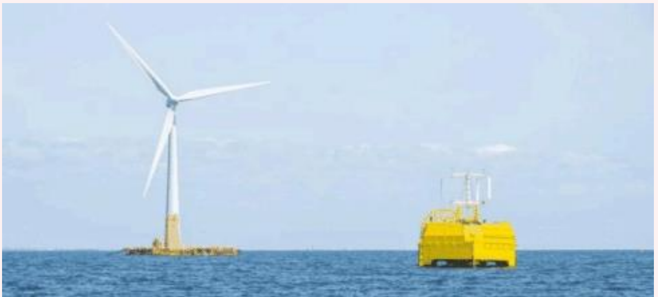
Figure 3. SeaLhyfe Offshore Hydrogen production integrated with a floating wind turbine
